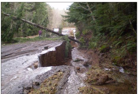
Fall and winter flooding has increased in western Washington over the past decade. Culvert capacity can be quickly exceeded during these events, leading to road failures and heavy erosion.
